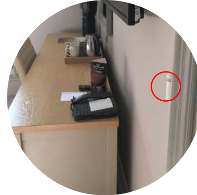
Monitoring room occupancy with discretely positioned motion sensors
